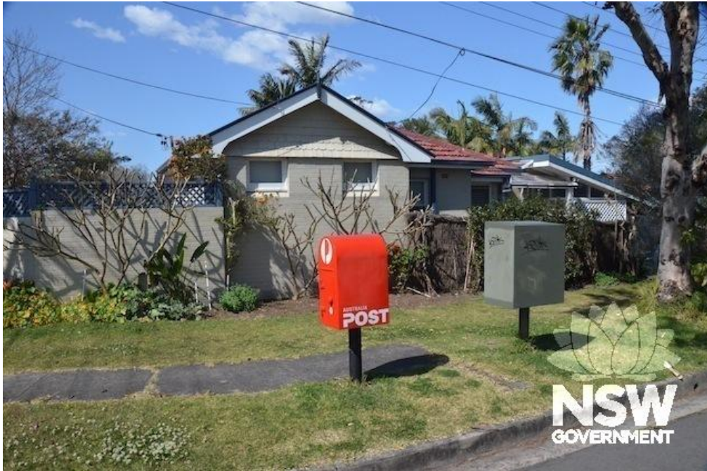
Figure 29: 30 Stuart Street, Longueville (Source: State Heritage Inventory database, “House”, 30 Stuart Street, Longueville, accessed via https://www.hms.heritage.nsw.gov.au/App/Item/ViewItem?itemId=1920194 )
