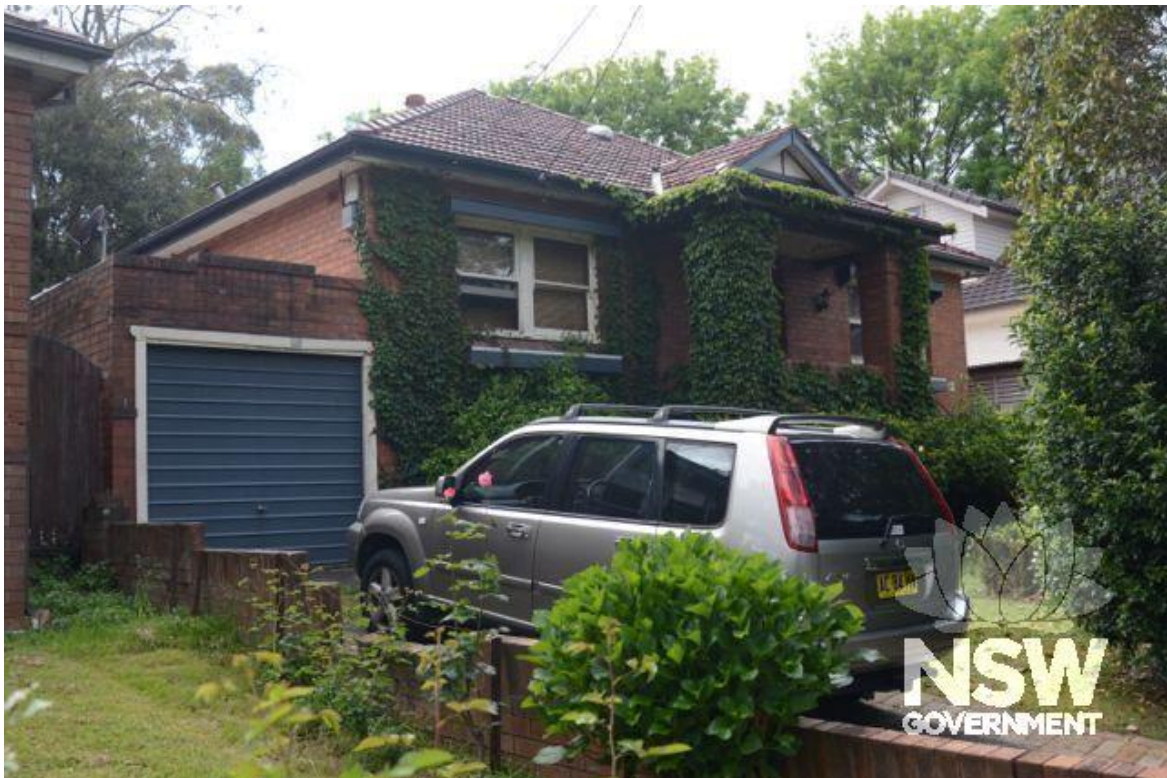
Figure 18: 3 Austin Crescent in 2013. (Source: State Heritage Inventory Database, "House", 3 Austin Crescent, Lane Cove, Heritage Item ID No. 5052822, accessed via https://www.hms.heritage.nsw.gov.au/App/Item/View/Item?itemId=1920294 )
