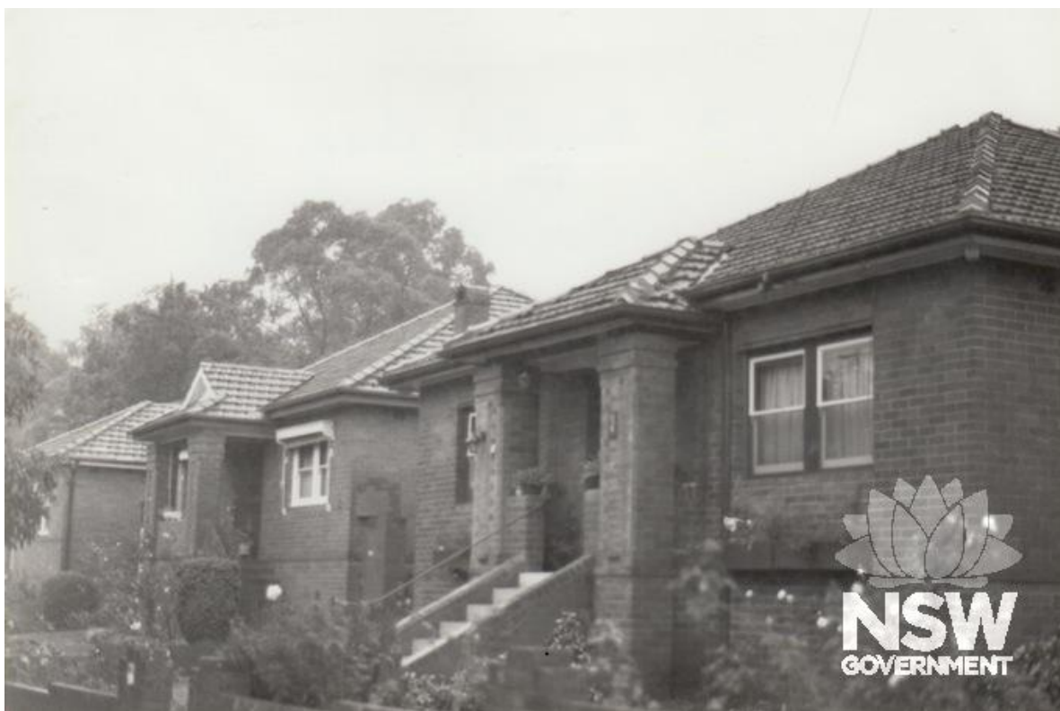
Figure 15: From left to right: no. 5, no. 3, and no.1 Austin Crescent in 1987, Lane Cove Council. (Source: NSW State Heritage Inventory form for listing 1920009, https://www.hms.heritage.nsw.gov.au/App/Item/ViewItem?itemId=1920009 , retrieved 16/04/2025)
